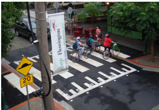
Figure 5 Raised crossing near on Pin Oak Crescent
