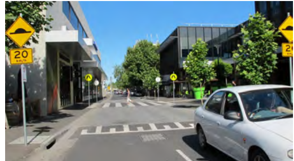
Figure 6 Raised crossing on Hall Street
